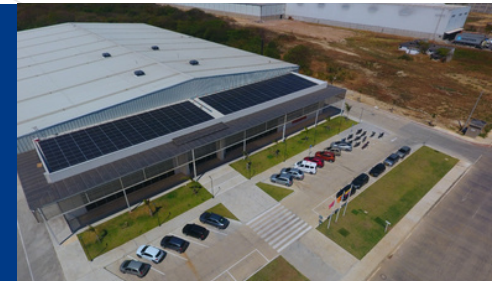
112 KwP Barranquilla Colombia
